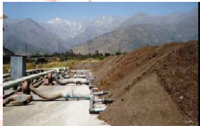
Fig 15. Aerated static pile compost
